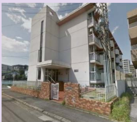
Exterior view of the dormitory
